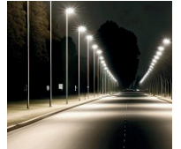
LED street lights
