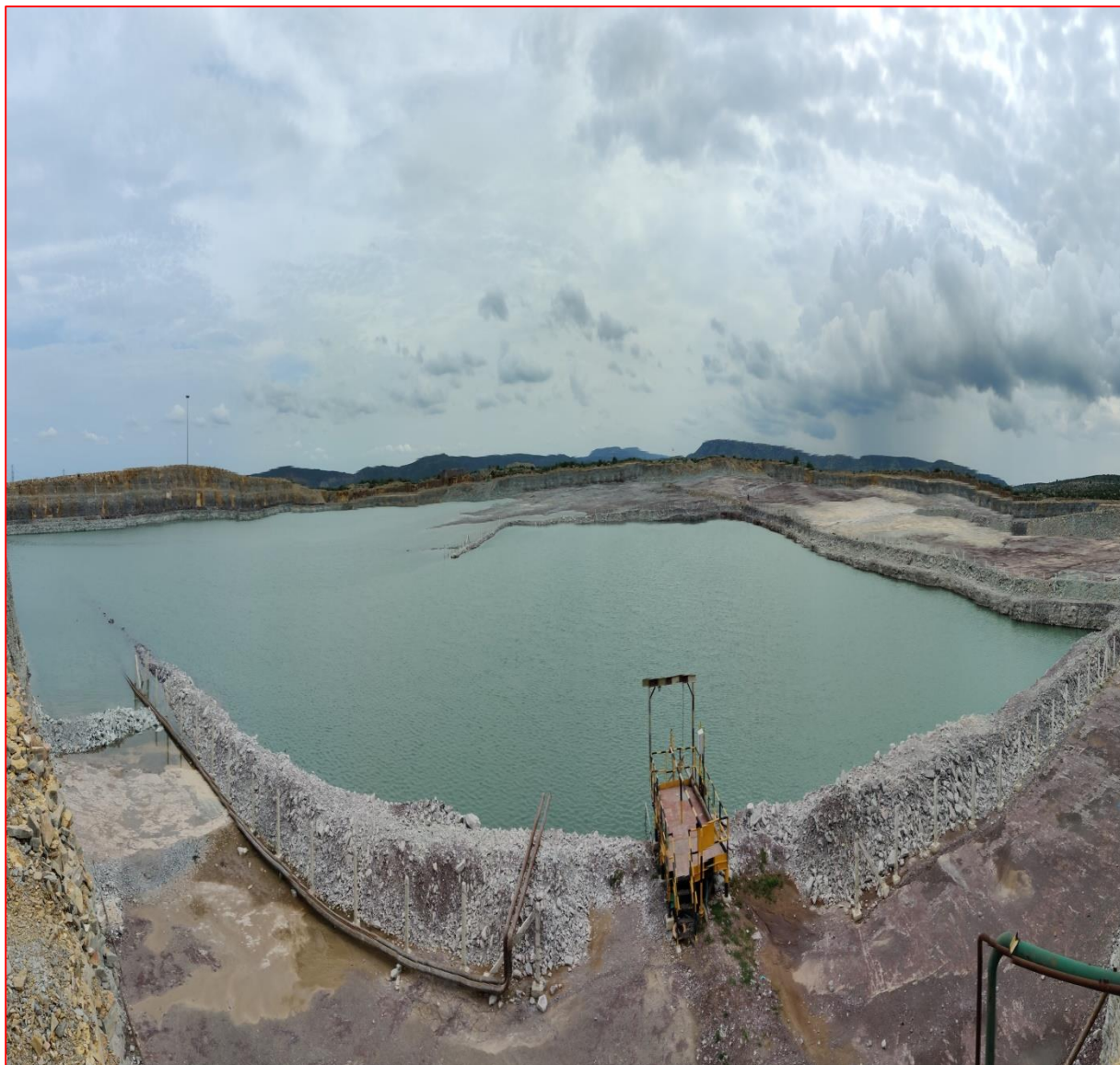
Rain Water Harvesting Pit
