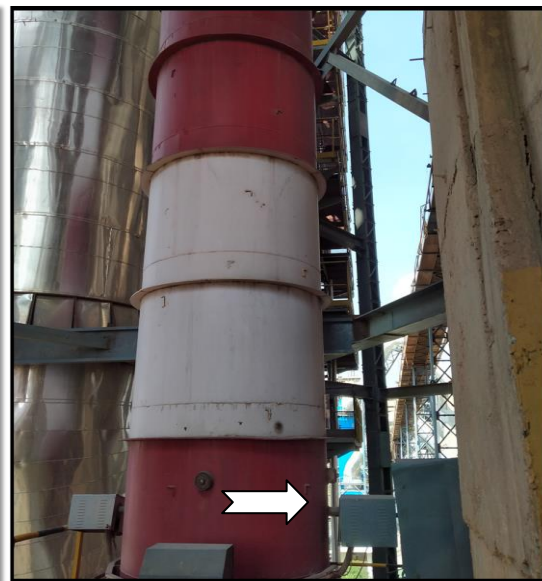
Coal Mill Stack
